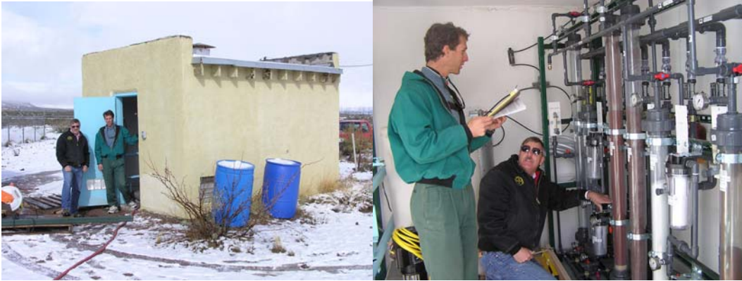
Figure 1. Socorro Springs Site and Pilot Equipment
